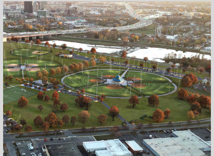
planned artificial turf infield upgrades, Kettering Field Sports Complex, Dayton OH
